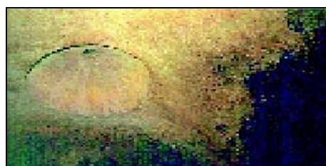
Figura 3.3 – Sofre incrustat a les parets internes del biodigestor [8]
