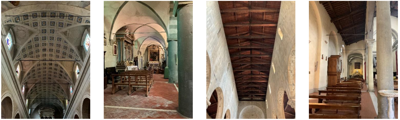
Figure 7. Examples of vault and roof structures. a) three-nave church, central nave vault ceiling; b) three-nave church, lateral nave vault ceiling; c) three-nave case, central nave timber trusses roof; and d) three-nave case, lateral nave sloping wood beams.
