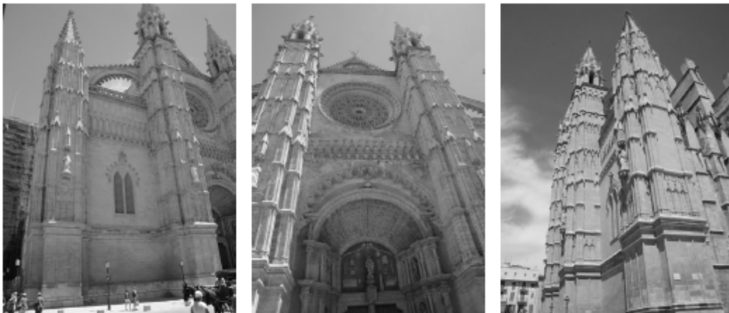
Figure 3.10 – Actual view of the West façade.
