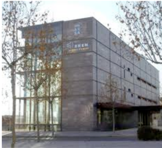
Figure 1.1 - Bioclimatic Building in Castile and Leon
