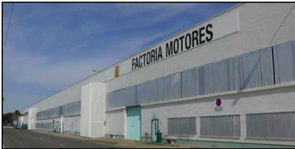
Figure 42- Renault Valladolid Engines plant. (Source: Renault Valladolid Engines)
