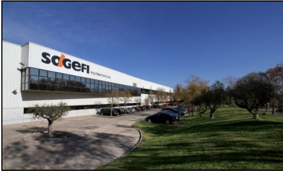
Figure 6- Sogefi Filtration Plant at Cerdanyola del Vallès. (Source: Mundorecambioy taller, 2012)
