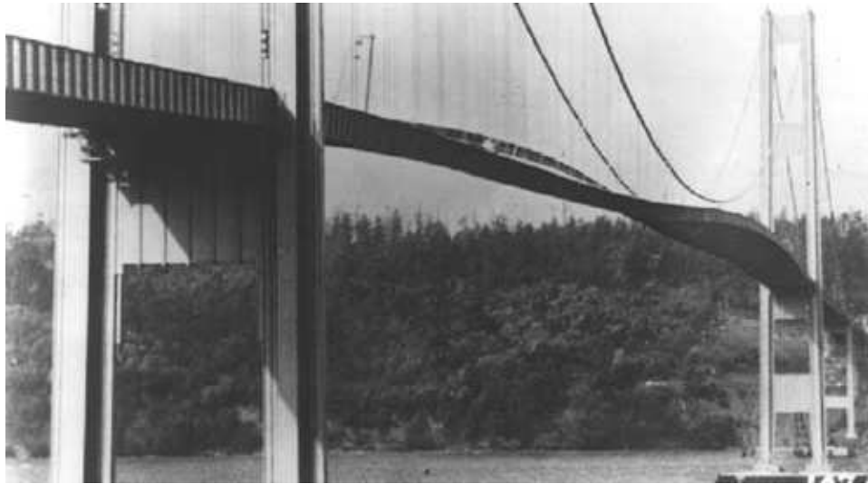
Figure 1.3 Aeroelastic instabilities of the Tacoma Narrows suspension bridge, U.S.A.
