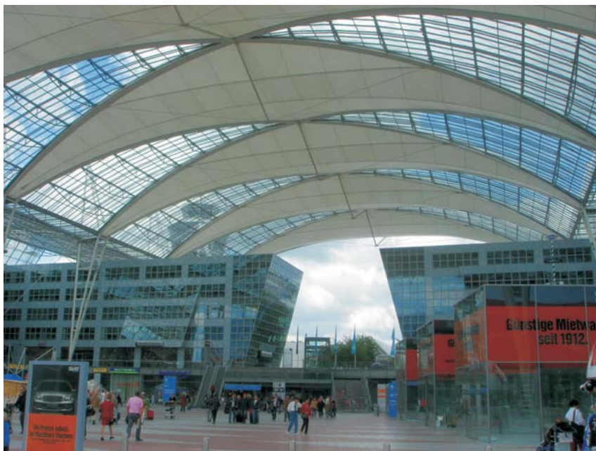
Figure 1.1 Membrane long span structure
