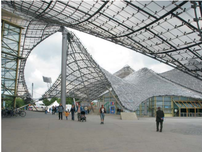
Figure 1.2 Prestressed membrane structure
