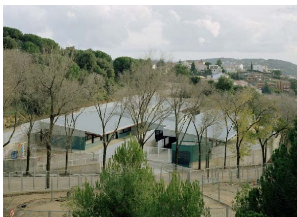
C.E.I.P. Can Matas, Sant Cugat, 2004, P. Pedrero.
