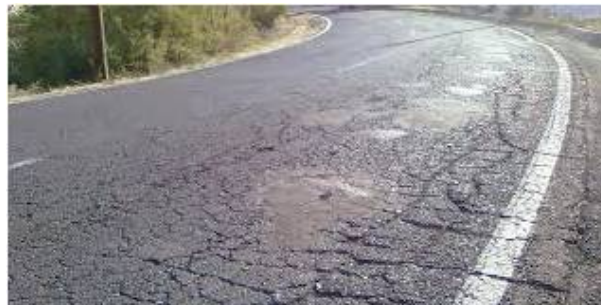
Figure 1.2: Filtrated water freezes and generates pressure in the crack.
