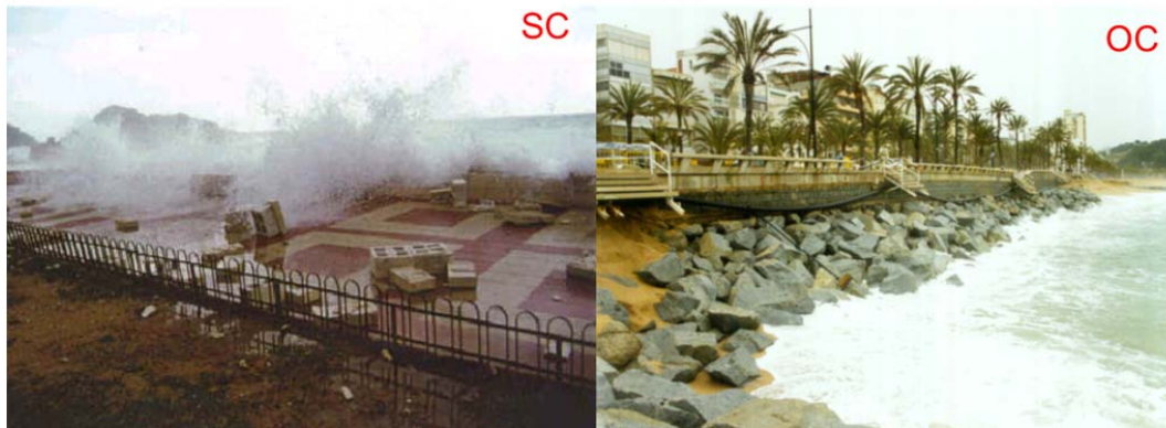
Figure 1. Extremes for survival conditions, affecting structural stability (left) and operational conditions, affecting the normal exploitation of the beach (right) for a beach promenade in the Catalan coast, NW Spanish Mediterranean.
