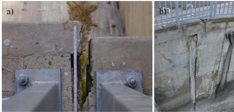
**Fig. 3.** a) Relative displacement in block 13-14 (downstream face) and b) joint 13 in the upstream face.
