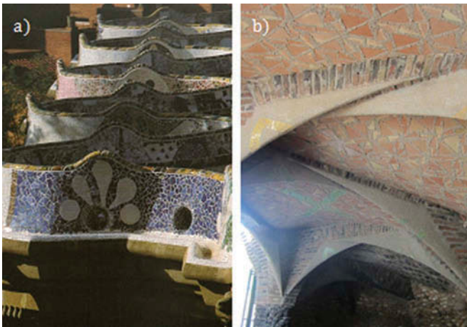
FIG. 7. (a) Parapet at the edge of the upper square of Parque Güell and (b) roof of the entrance porch leading into the crypt of the Colonia Güell (2011). © (a) J. Bergós. Reproduced by permission of J. Bergós. Permission to reuse must be obtained from the rightsholder.
