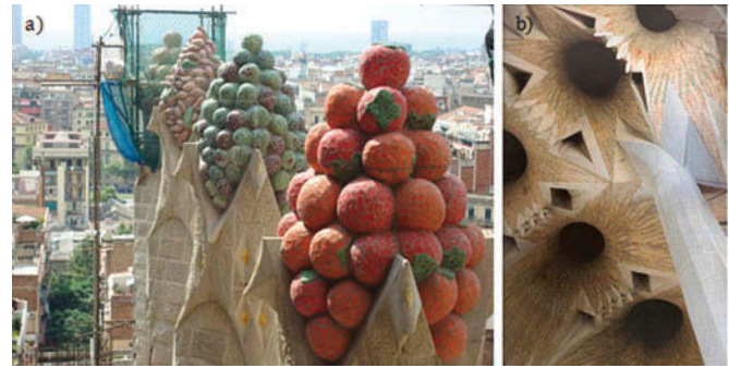
FIG. 15. (a) Pinnacles of the windows in the building (2011), and (b) hyperboloids in the ceiling of the building decorated with Murano glass. © (a) J. Bonet. Reproduced by permission J. Bonet. Permission to reuse must be obtained from the rightsholder.
