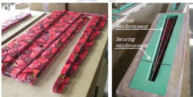
FIG. 18. (a) Preparation of trencadis glass before its assembly in the mold, and (b) Assembly of trencadis and reinforcements in the mold. © (a) Archivo Histórico De La Basílica De La Sagrada Familia. Reproduced by permission of Archivo Histórico De La Basílica De La Sagrada Familia. Permission to reuse must be obtained from the rightsholder.
