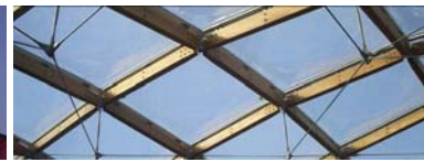
Fig. 13 Alnwick Gardens Visitor Centre de Northumberland, Hightex.
