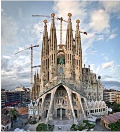
Fig. 12. Photograph of the exterior of the building.
