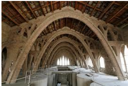
Fig. 9. Photography of the interior of the building.
