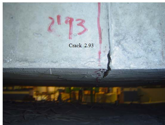
Photograph3. Cracking Location (Fourth stretch)
