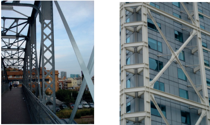
Figure 5. Examples of structures containing Saint Andrew's crosses. PONS (2014).
