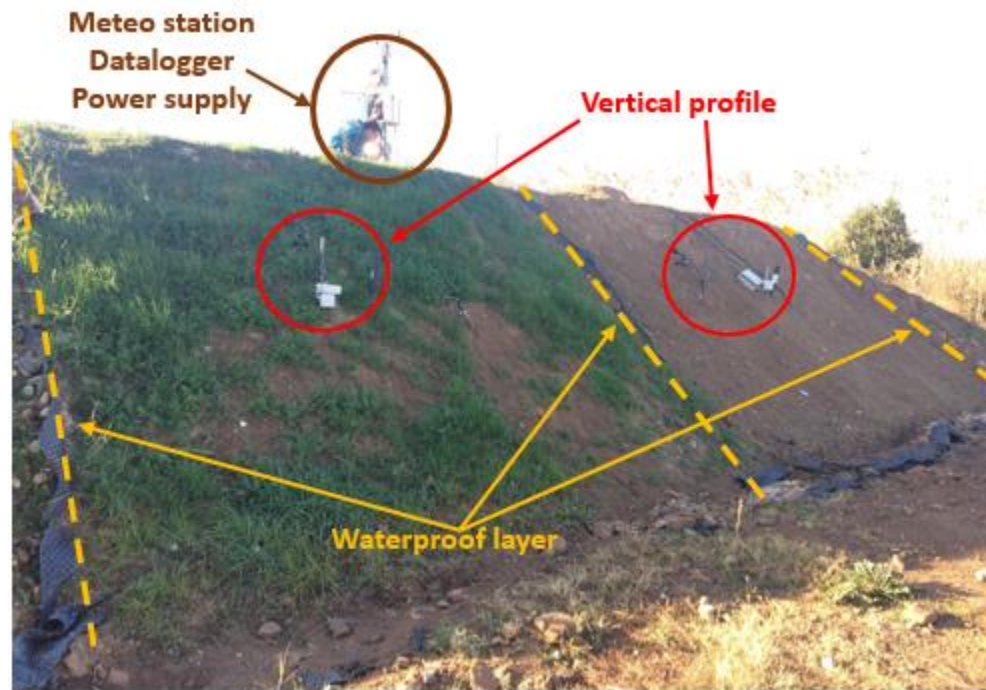
Figure 2.3: Photograph of the embankment after installation of the sensors looking towards the North slope.
