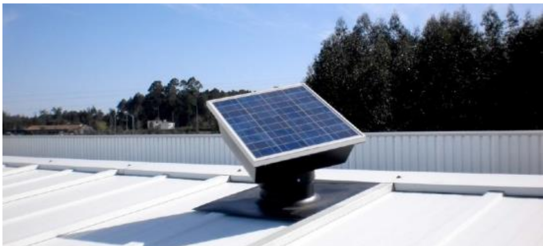
Figura 43. Extractor solar per as cobertes
