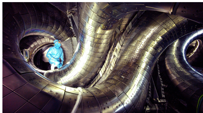
Figure 5: Inside the LHD reactor [4]
