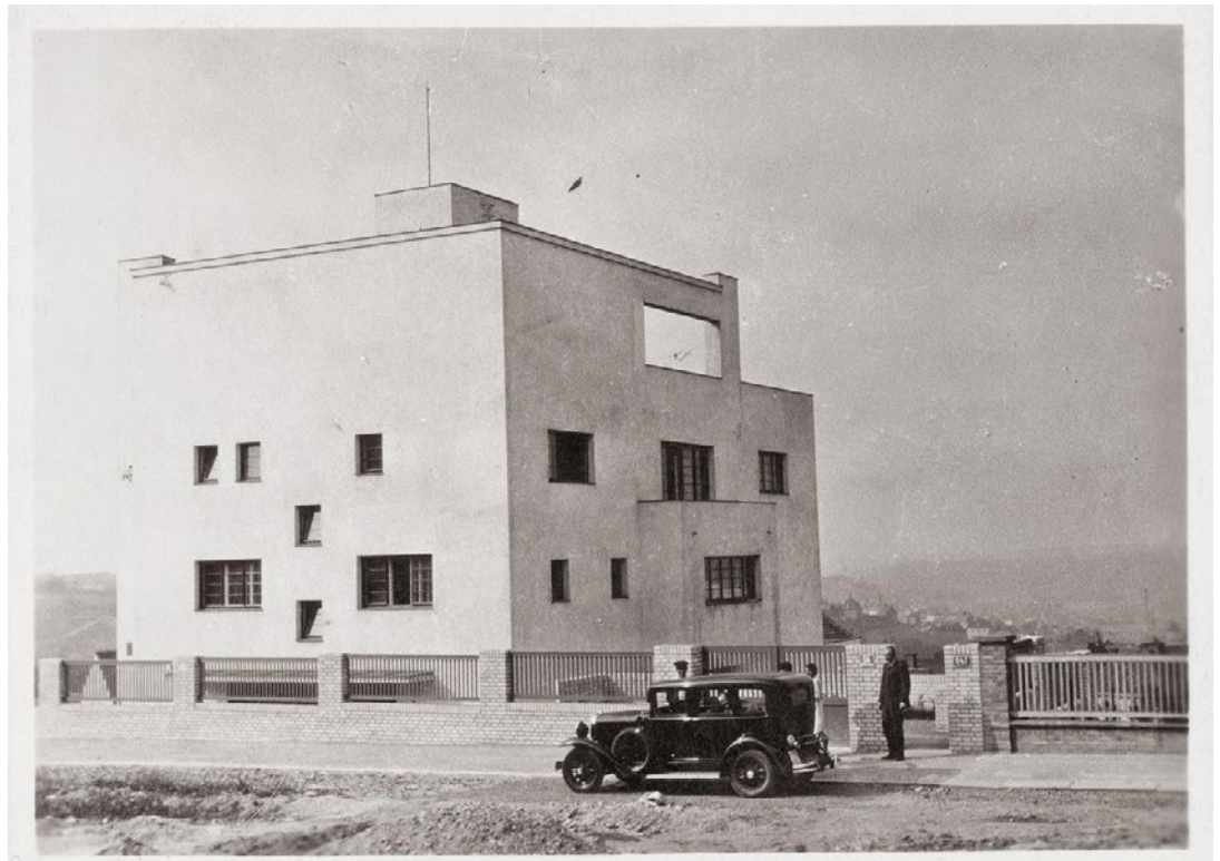
Image 16. Exterior view of the Müller house, Vienna. Image obtained from: https://rjaviarsar.wordpress.com/2014/12/22/la-villa-muller-1928-1930_-_adolf-loos/
