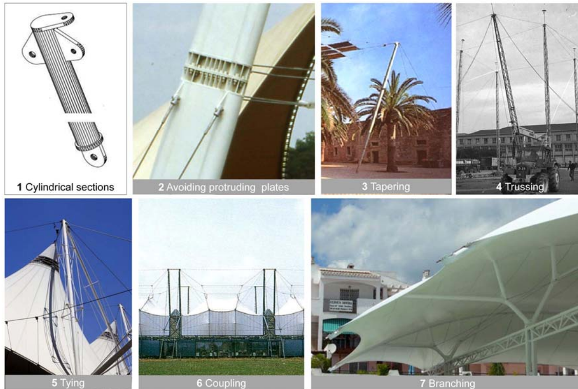
Figure 4: the masts accept different strategies to cope with over-dimensioning imposed by buckling on such long elements.
