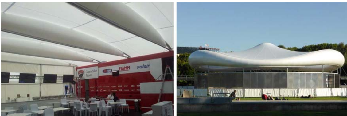
Figure 10: Maco Technology, 2014: The Ducati hospitality tent is also based on Tensairity beams which span 12 m.
