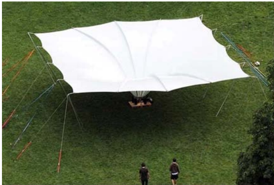
Figure 12: Institute of Building Structures and Structural Design, 2011: an innovative membrane structure for a schoolyard roofing comprises 7.5 m long, elastically-bent fiberglass rods (in pockets) for the pre-stressing of the membrane.
