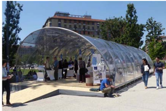
Figure 13: C.Mazzola & A.Zanelli with Form TL and Canobbio, 2019: "TemporActive Pavilion", an ultra-lightweight temporary structure consisting of bending active GFRP arches, a restraining system made of stainless steel cables, and an ETFE translucent membrane envelope.
