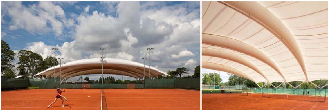
Figures 8,9: G.Stowell, Architect with form TL and Canobbio, 2010: The sports canopy for the National Tennis Centre, London is a wide-span membrane which consists of five Tensairity beams with membrane panels in between.
