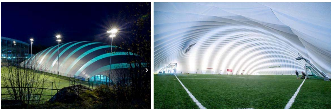
Figures 3,4: Canobbio Textile Engineering, 2016: Air hall for the Helsingin Jalgpalloklub football team field, Helsinki
