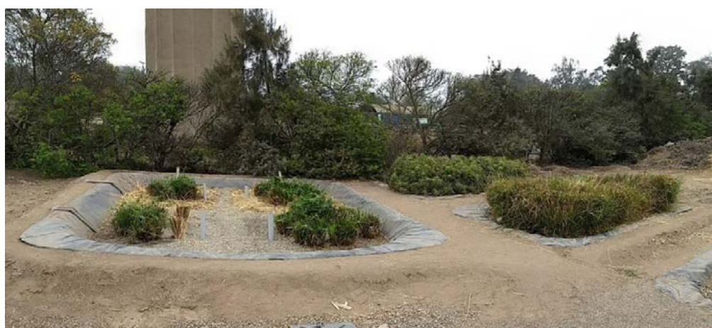
Figure 1. French System of UNALM. Left: 1 st stage (French cell); Right: 2 nd stage (vertical flow subsurface wetlands)
