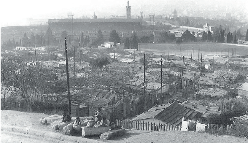
Figure 3. Settlement in Monjuïc (1967). Source: Camino et al. (2011)
