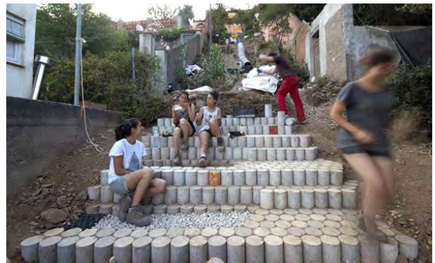
Figure 1. ‘Ruta Ringo Rango’ academic project, built by students of PUD Studio with support from local community and the municipality of Sant Cugat del Vallès, Barcelona, 2015.
