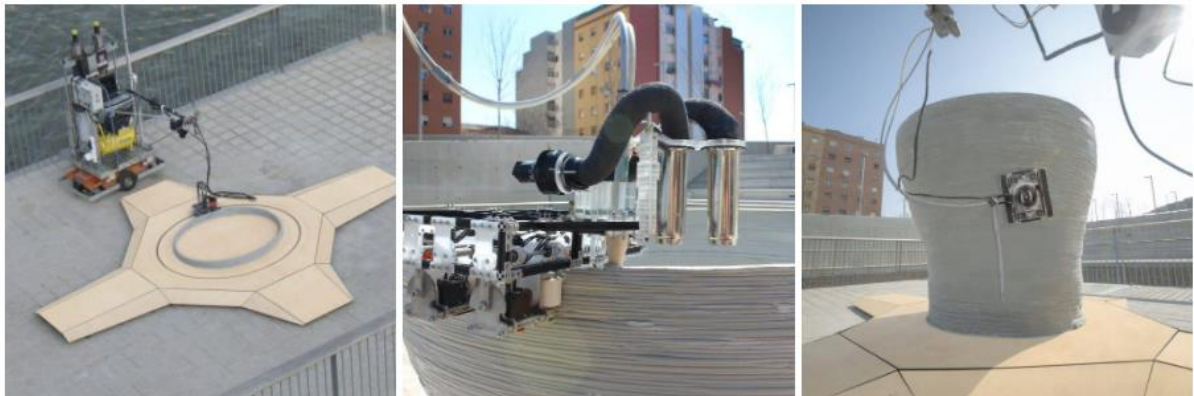
Figura 23:1, 2 y 3 Minibuilders del Institute for advanced Architecture of Catalonia
