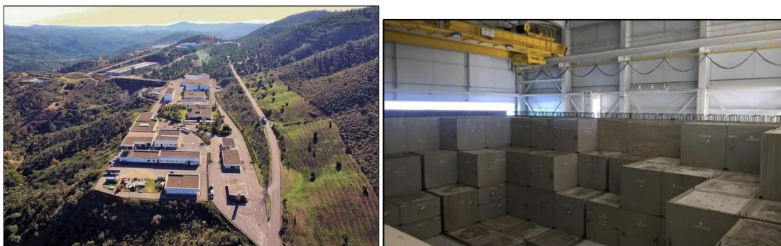
Figure 1.1. CA El Cabril facilities and the storage cell of the nuclear waste.
