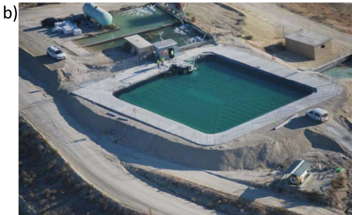
151 Figure 1. Schematic view showing: a) the integration of the solar pond with the 152 mineral flotation process in Solvay Minerals facilities and b) view of the 500 m 2 153 solar pond at Solvay Minerales facilities (Granada, Spain)
