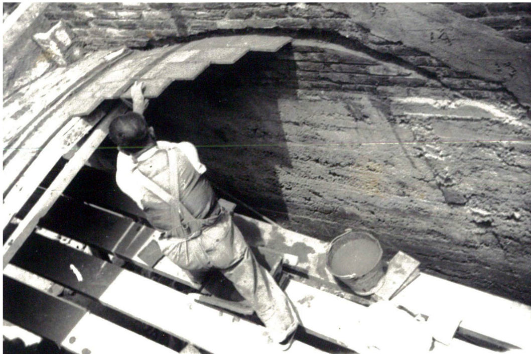
Fig. 1. Construction of a tile vault [8].
