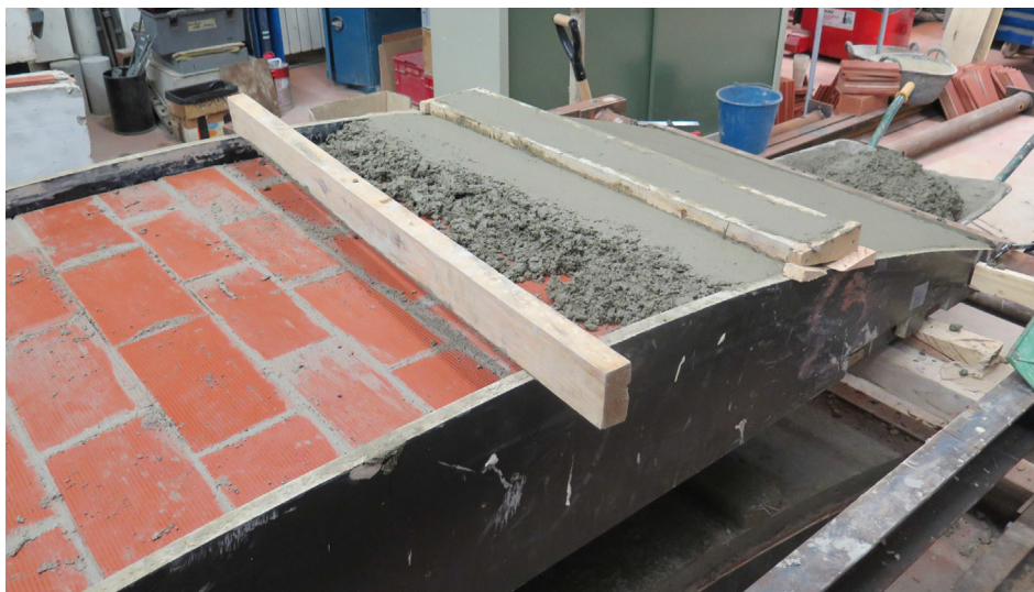
Fig. 4. Construction of the tile-concrete composite barrel vaults.
