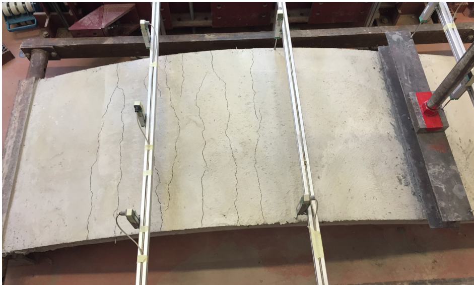
Fig. 25. Cracks on the extrados of the composite barrel vault 4.
