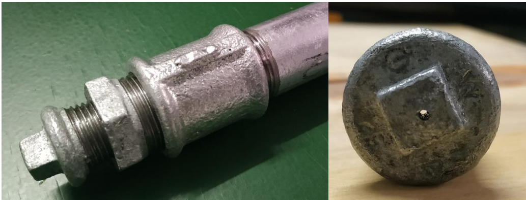
Figura 46: Broquet i part final del fuset
