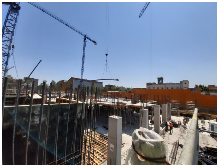
Figure 11 View from the street ((Universitat Politecnica de Catalunya, 2021)
