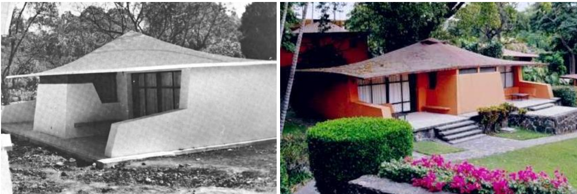
Figure 18. In the left the original inverted umbrella roof can be observed, meanwhile in the right an opening can be noticed because the temperature was hot inside the bungalows of Casino de la Selva.
