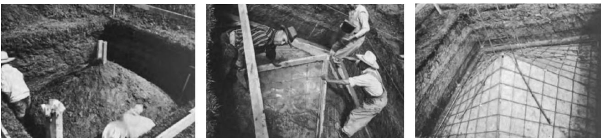
Figure 14. Inverted umbrella footing construction process.
