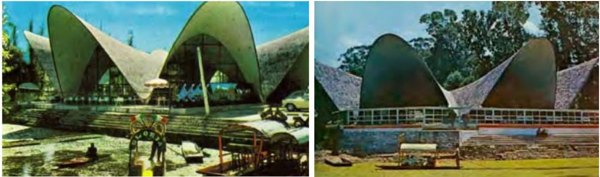
Figure 39. Water level changes and additions at the exterior of the restaurant.
