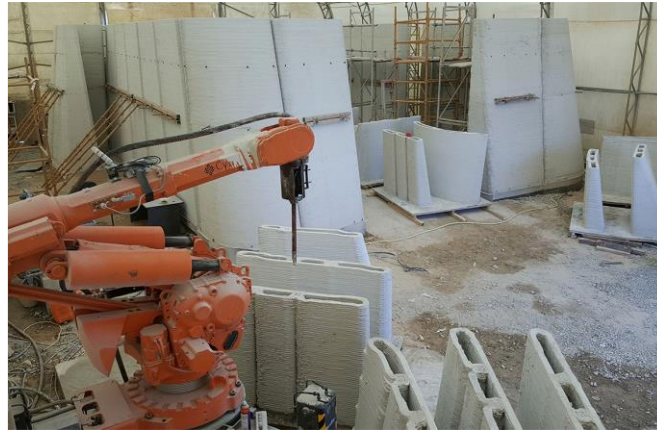
Figure 19 3D printing by CyBe [37]
