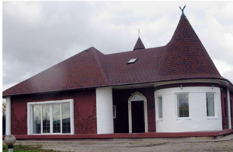
Figure 22 3D printing by Spetsavia [40]
