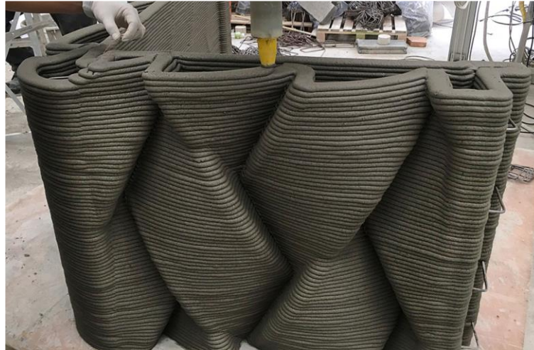
Figure 29 3D printing by SCG [48]
