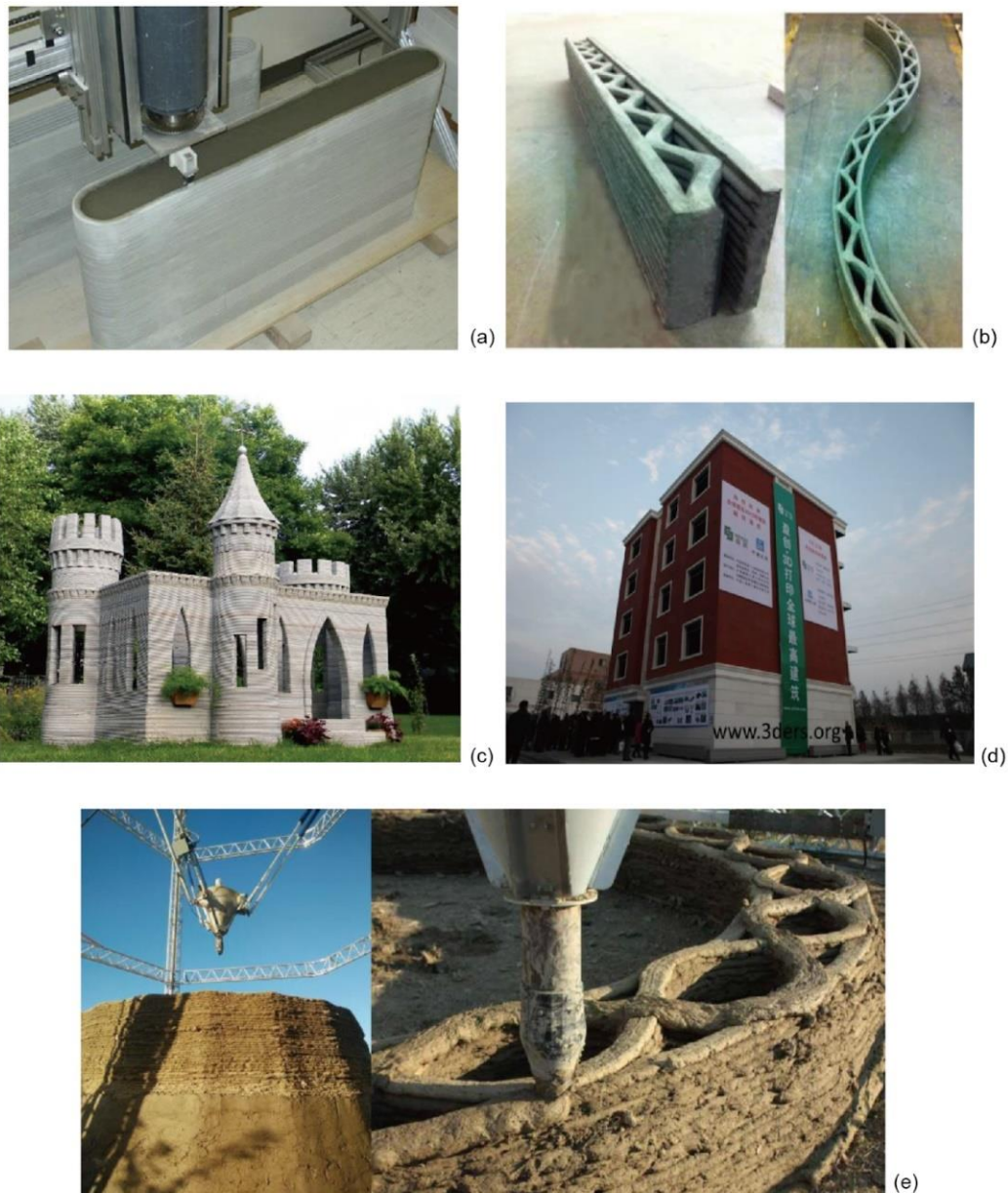
Figure 45 Examples of full-scale builds from contour crafting printing [103]
