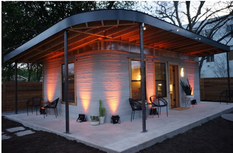
Figure 24 3D printing by ICON [43]
