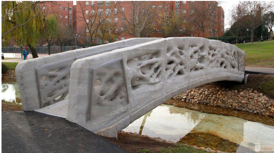
Figure 13 Pedestrian bridge constructed by a D-Shape 3D printer [24]
