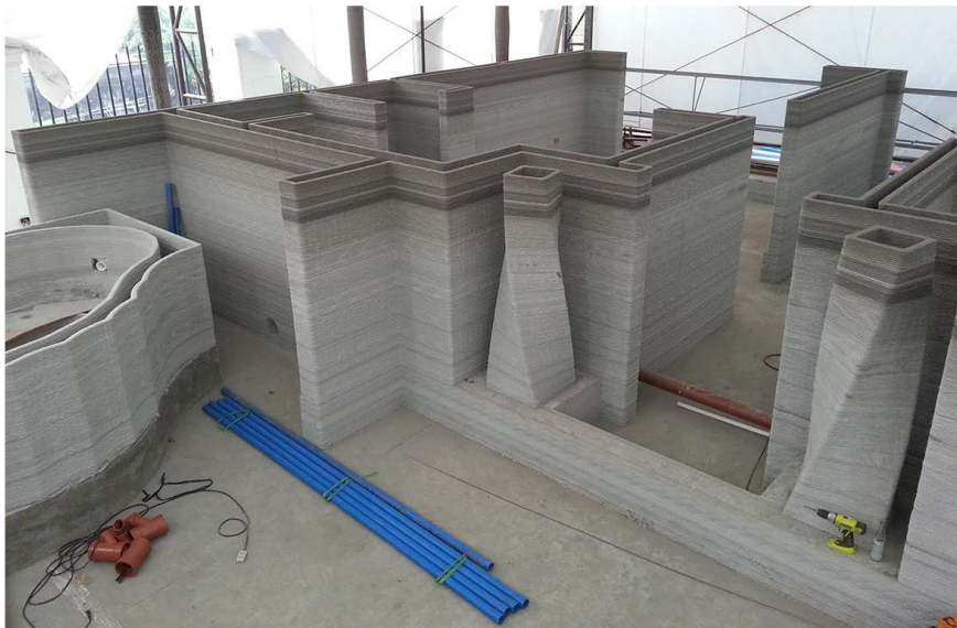
Figure 18 3D printed hotel Room [35]
