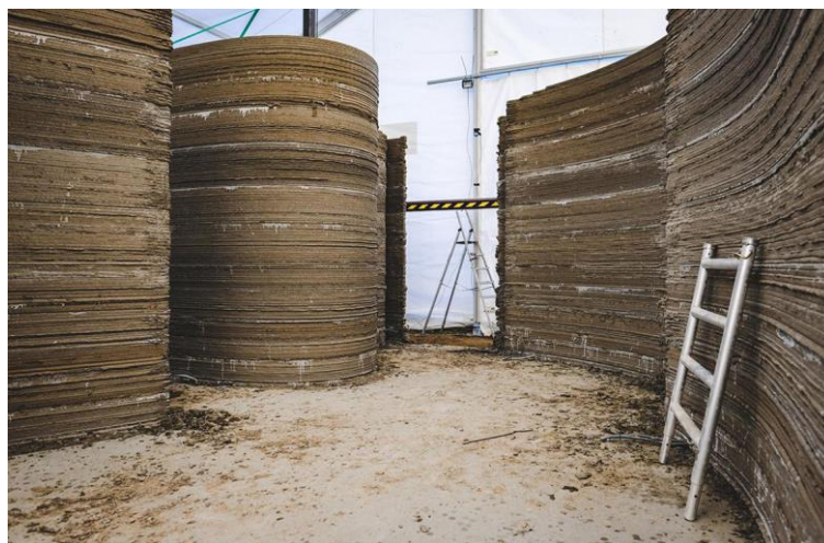
Figure 21 3D printing by 3D PrintHuset [39]
