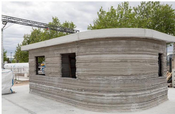
Figure 25 3D printing by Be More 3D [44]
