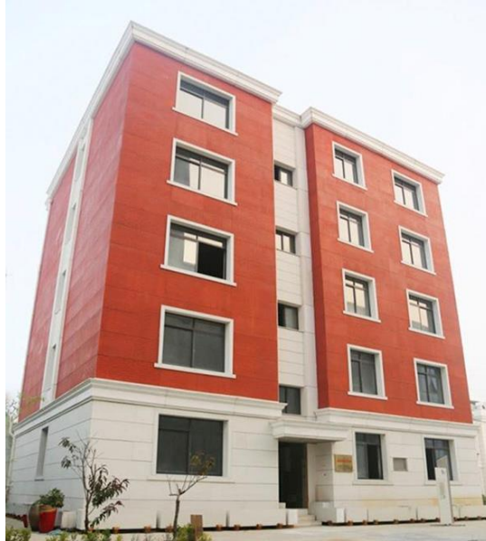
Figure 15 3D printed multi-story apartment building [34]
