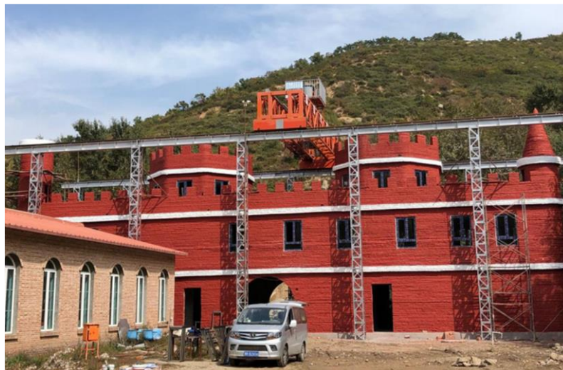
Figure 23 3D printing by HuaShang Tengda [41]
