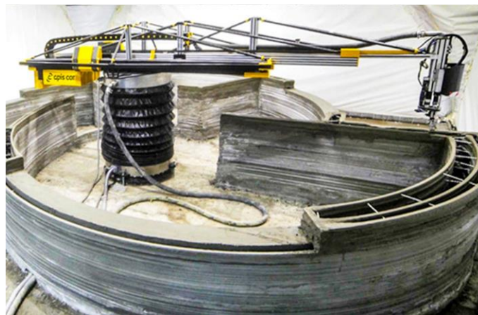
Figure 20 3D printing by Apis Cor [38]
