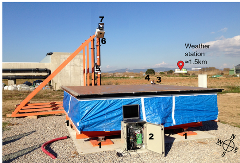
Fig. 1. Overview of the field test: 1) steel structure, load cells and coupling; 2) data recording system; 3) anemometer; 4) two VP3 sensors to measure relative humidity, temperature and vapor pressure; 5) support structure; 6) digital camera; 7) IR120 infrared remote temperature sensor.
