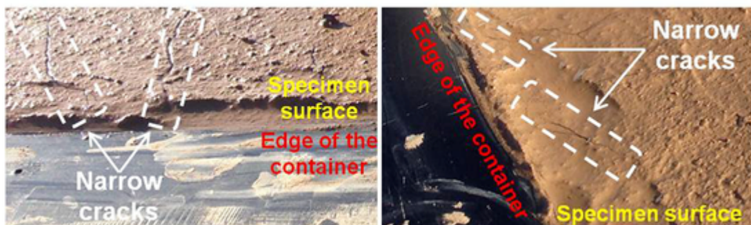
Fig. 10. Thin cracks formed close to the lateral walls of the container at the start of the test.
