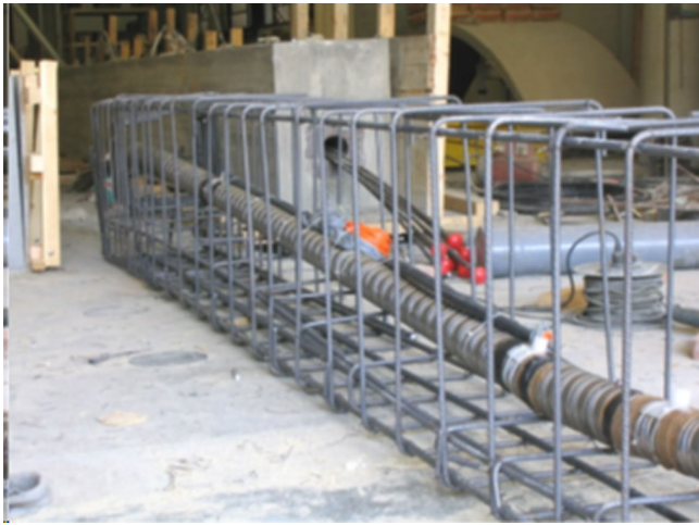
FIGURE 7 Monitoring of the strands of the post-tensioned concrete beam tested, 16
