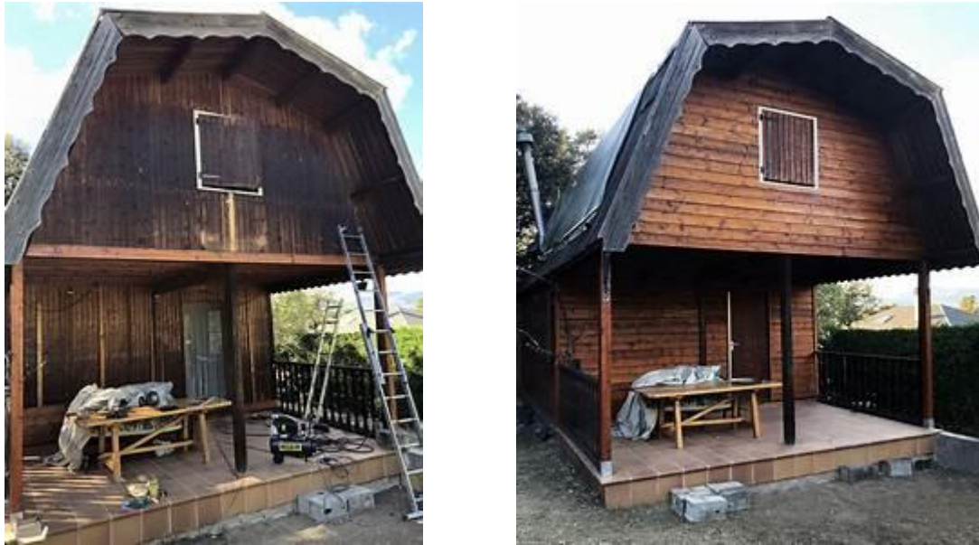
Figure 2.1 Degradation of the color of the pine wood of the façade and replacement by new pine slats Source: https://www.mcmcasas.com/project/fachada-madera-2/
