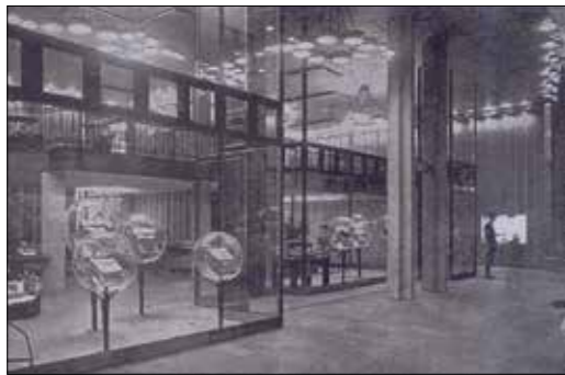
Photos taken from the publication of the project of the Hispano Olivetti Building, Barcelona, 1964
