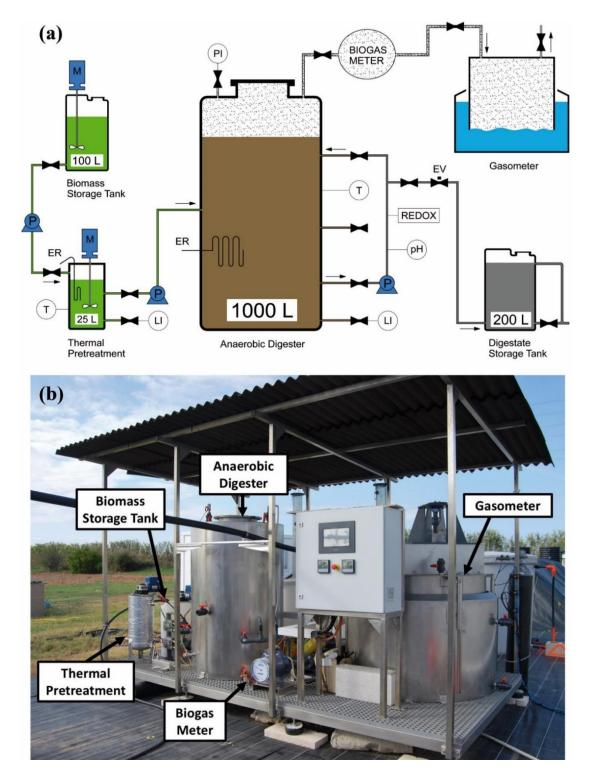
**Figure 2.** (a) Diagram of the anaerobic digestion plant. Mixers (M), pumps (P), electrical resistances (ER) and electrovalves (EV) are indicated in the figure, as well as the temperature (T), liquid level (LI), pressure (PI), redox and pH sensors. (b) Image of the anaerobic digestion plant.
