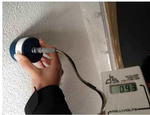
Figure 2. Use of the emissometer to determine the wall surface emissivity (0.93).
