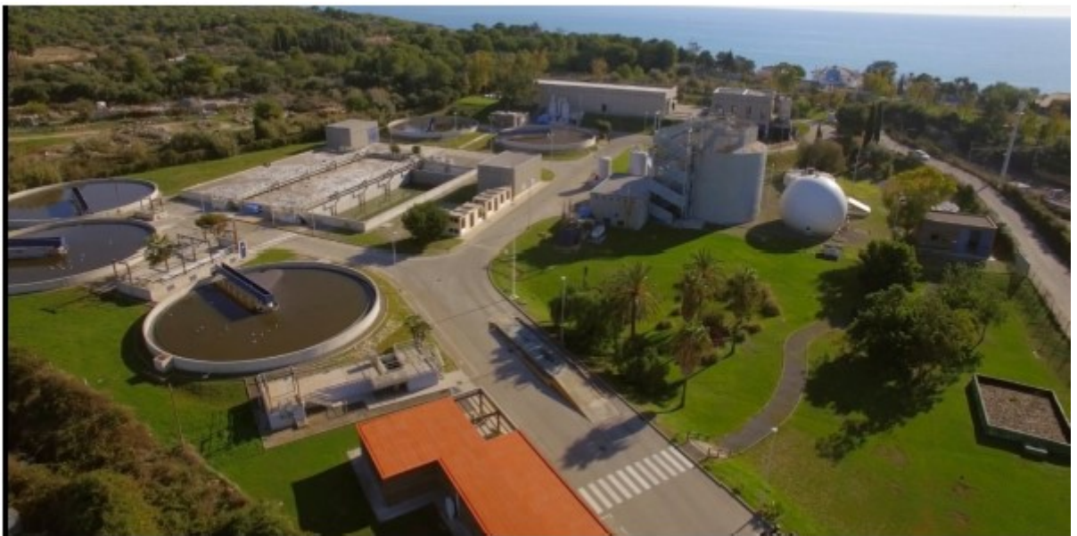
fig. 8 Aerial view of Vilanova WWTP
