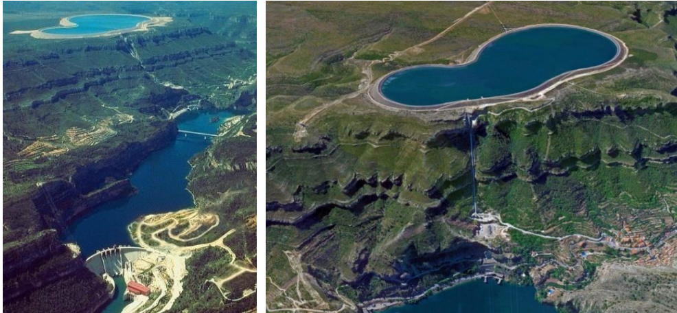
Figure 2. La Muela pumped hydroelectric energy storage power plant. (Source: www.nsenenergybusiness.com)
