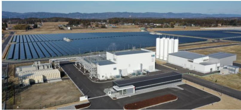
Figure 8. FH2R 10 MW hydrogen production plant in Fukushima. (Source https://fuelcellworks.com/ )
