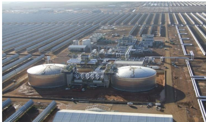
Figure 7. Manchasol & Extresol Solar Thermal Complex (Source: CSP focus)
