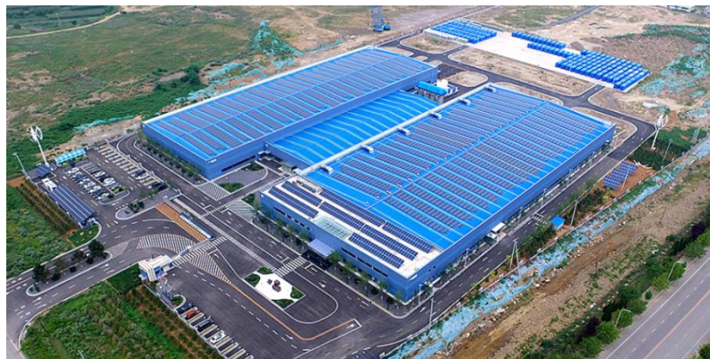
Figure 11. The world's largest VRF battery: 200MW/800MWh in Dalian, China. (Source: Rongkepower)
