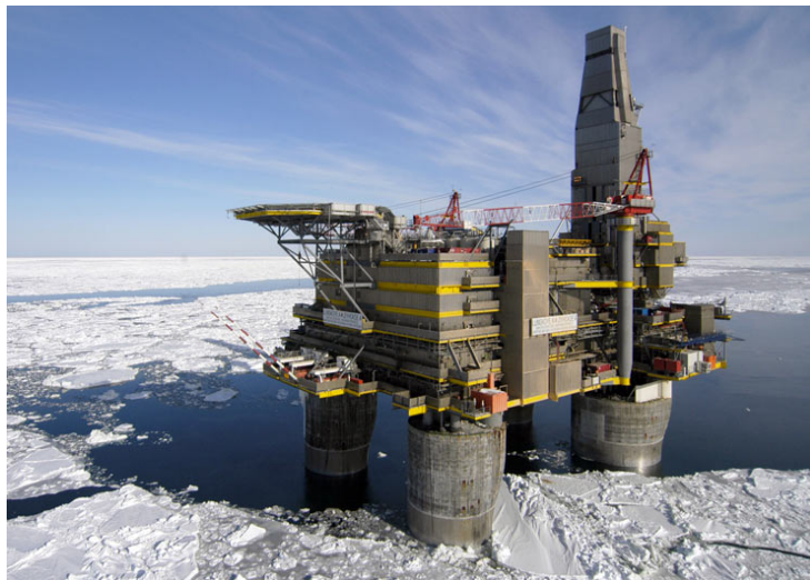
Figure 1: Gravity base structure “Sakhalin II” in the arctic region (source: http://gazprom-sh.nl )
