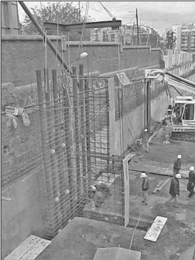
Fig. 7. Placing the reinforcement cage with straight ducts for post-tensioned tendons
