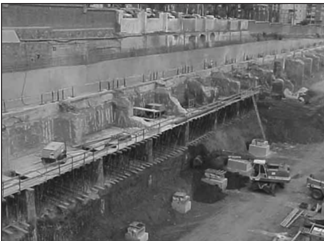
Fig. 8. Buttressed diaphragm wall after excavation and during construction of floor slabs
