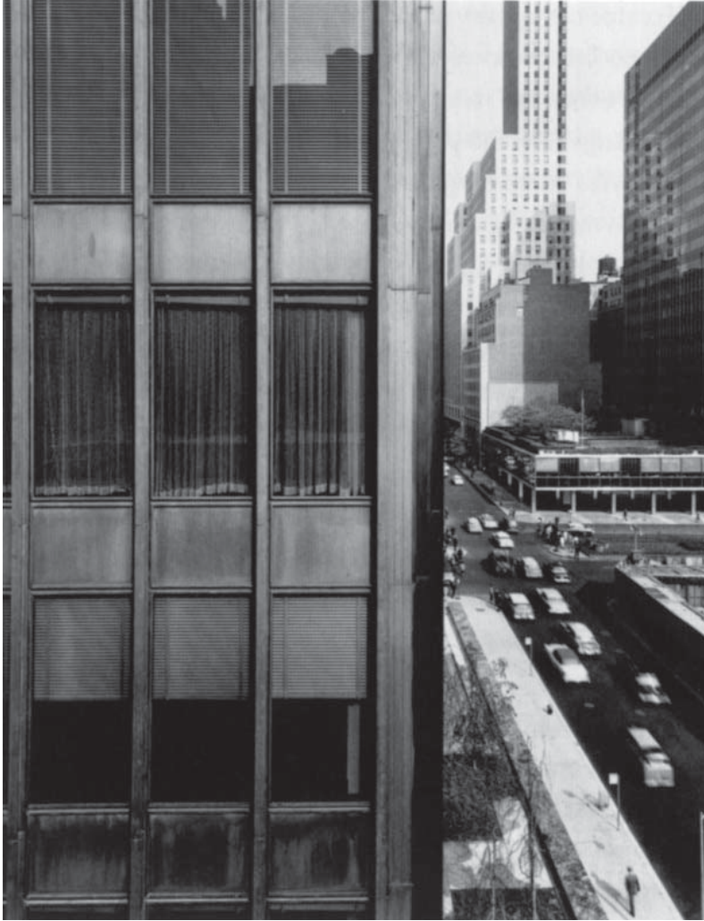
En primer plano, la fachada de bronce del Seagram. A la derecha la calle 53, la Lever House, y de fondo el Du Mont building, 1931 (162m). Foreground, Seagram bronze facade. Lever House on the right, 53th street, and the Du Mont building at the background, 1931 (162m).
