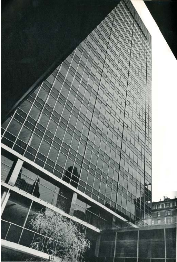
Vista desde el patio. View from the courtyard.
