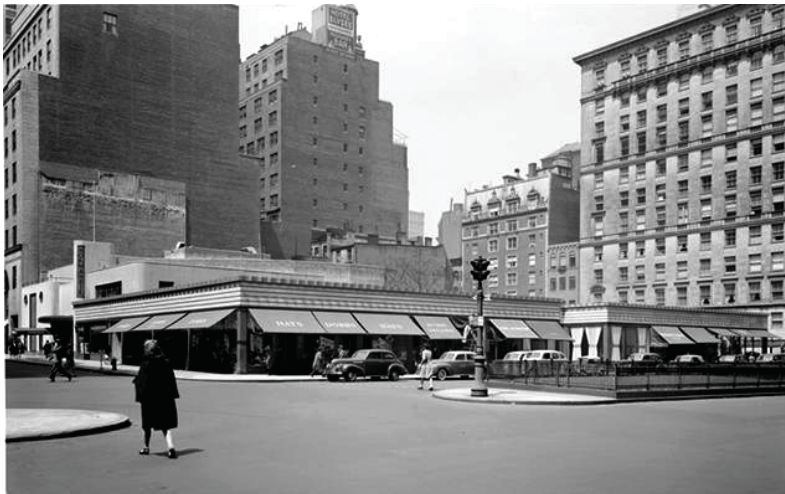
Edificio tax-payer de Rosario Candela, entre las calles 53 y 54, 1944. Tax-payer building by Rosario Candela, between 53th and 54th streets, 1944.
