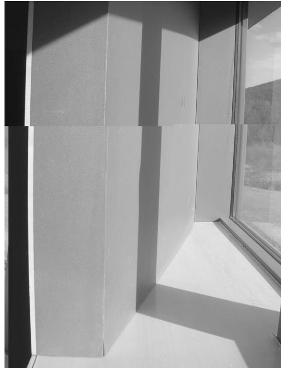
Figure 7. Absorption panel on the south-oriented façade.
