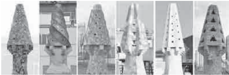
Fig. 1. Palau Güell Chimney Stacks examples
