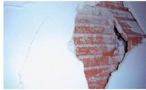
Detail view of an area of the crack: the plaster has separated cleanly from the ceramic brick without existing prior grip
