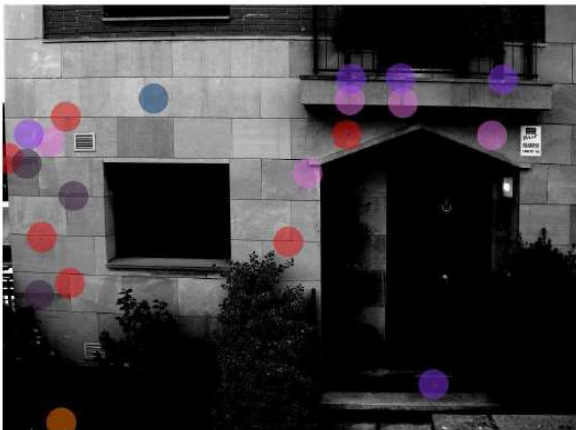
Figure 23 – Planimetry based on photographs to facilitate identification, census and classification of anomalies detected in the natural stone façade placated by a group of single houses
