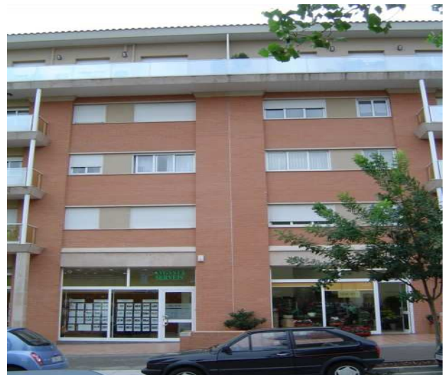
Figure 15 – View photo of a set of newly constructed residential buildings in urban peripheries
