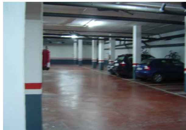
Figure 17 – General view photo of underground parking of vehicles in an apartment building
