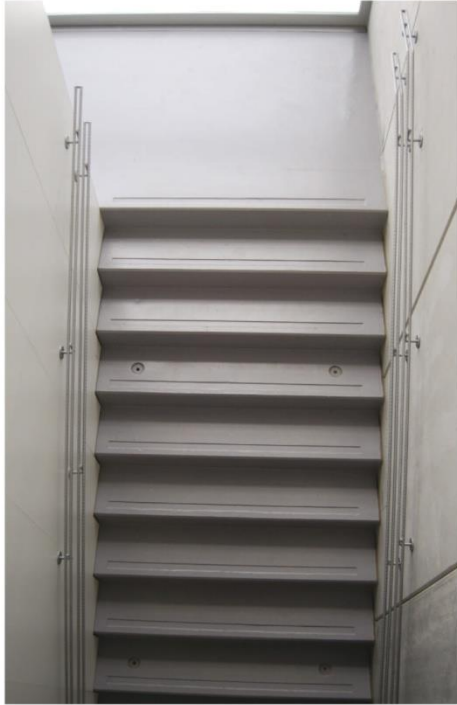
ESCALERAS_prefabricas on site
