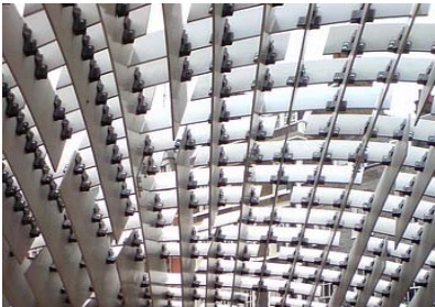
Ten Pavilion - Alan Dempsey i Alvin Huang : Plaques de GRC de 13 mm Ref: http://www.core.form-ula.com/2007/11/05/drl-ten-pavilion-design-competition-2007/
