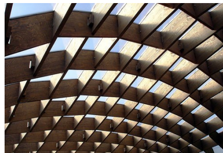
Serpentine - A. Siza i E. Souto de Moura : Estructura reticular Ref: http://museocactaceos.blogspot.com/2008/04/siza-serpentine-gallery_20.html Llibre "Serpentine Gallery Pavilion 2005 designed by Alvaro Siza Eduardo Souto de Moura"
