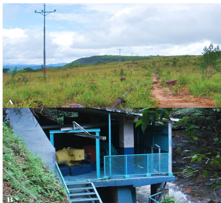
Figure 3. (A) Power and water lines from Apacairo; (B) MHP operations center in Kavanayén
