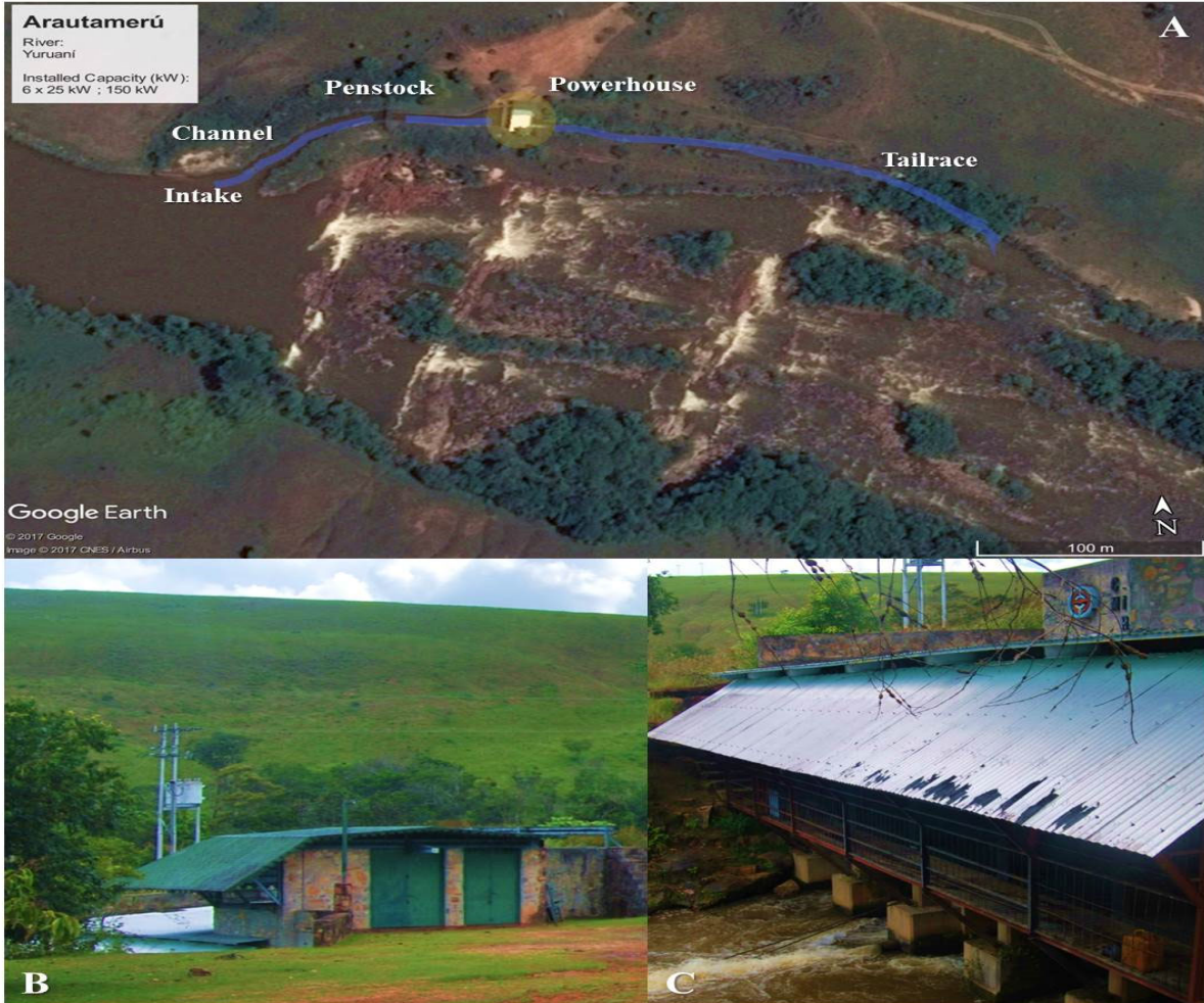
Figure 5. (A) Satellite image of Arajamerú micro-central (B) Powerhouse (C) Drain
